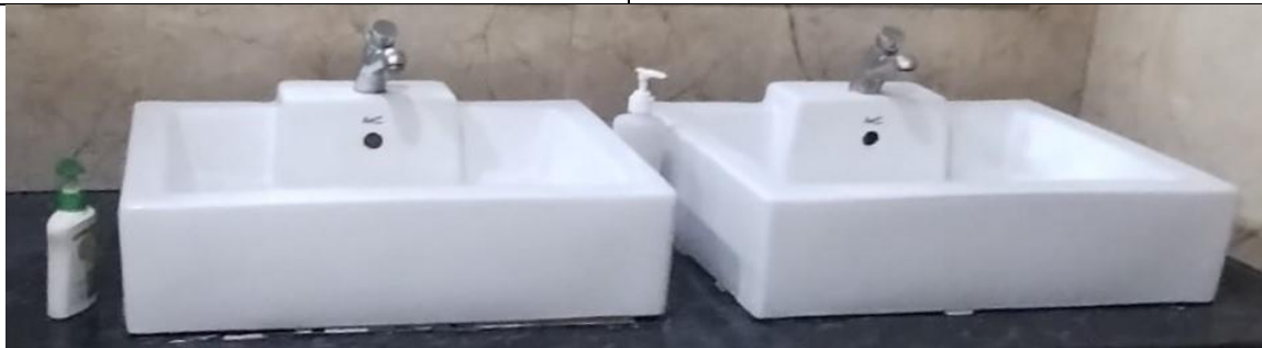
Upgraded version of Pressmatic Water Tap for minimizing water wastage
